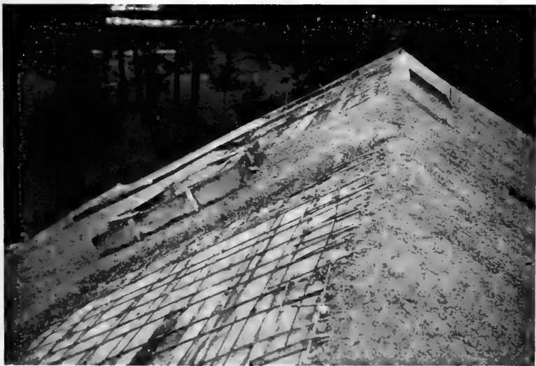
8—The Roof, its First Coat of Concrete and the Reinforcing Rods in Place
